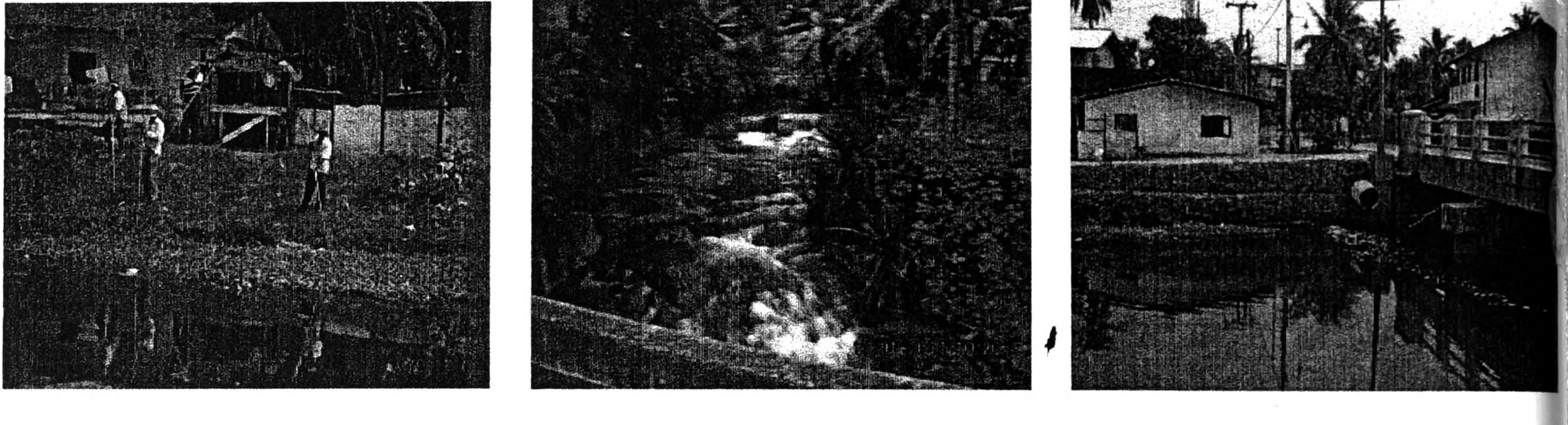
Plates showing condition in Lunawa lagoon system
